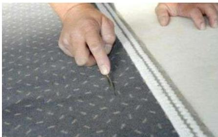
The seam along the marked channel line can be cut using a pile channel cutter or a sharp hook blade.
